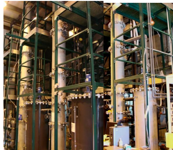
250 kW Chilled Ammonia Process Mini-pilot System
